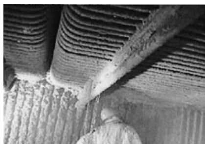
Photo 1 Cleaning work of incineration boiler system
