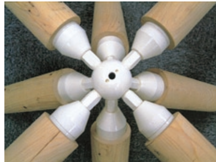
Photo 1 Joint detail
