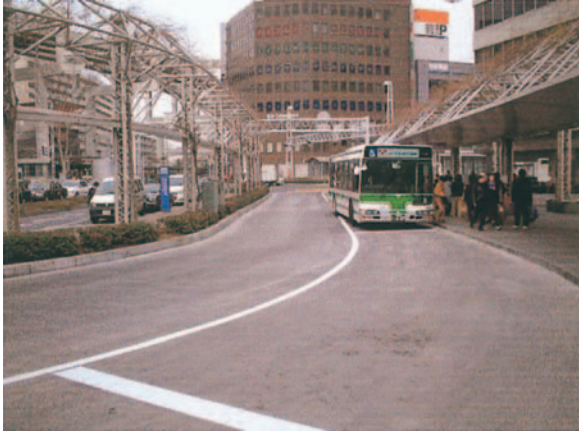
Photo 5 Asphalt-slag complexed pavement
