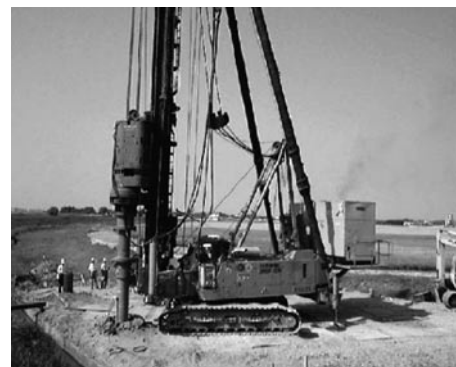
Photo 3 Construction of tsubasa pile using pile driver
