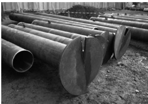
Photo 1 Screw pile, tsubasa pile
