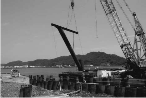
Photo 4 Strutted frame quay-wall structure
