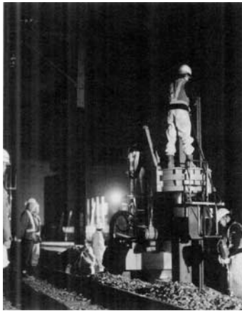
Photo 2 H-shaped steel sheet pile(K-domeru)
