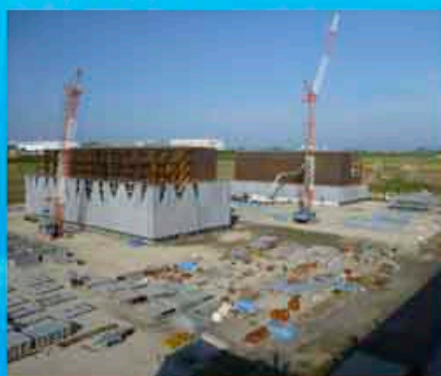
釜石港湾口防波堤
