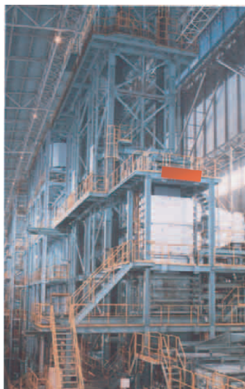
Photo 1 Fukuyama No.3 continuous annealing line equipped with water quenching (WQ-CAL) 1)
