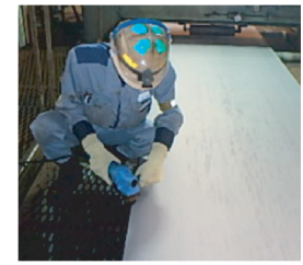
(b) Removal of defects
