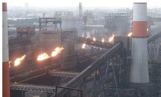
Photo 1 Operational status of actual machine
