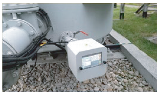
Photo 2 Appearance of continuous monitoring device for dissolved gas in insulating oil 2)
