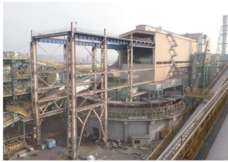
(a) Appearance of No.3 SP building
