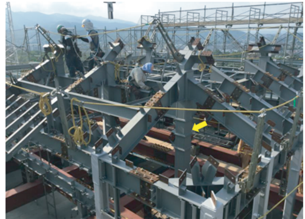
Photo 1 Steel frame of Kumamoto Castle's large keep (Arrow points to box column made with ultra-narrow-gap J-STAR™ welding technology)
