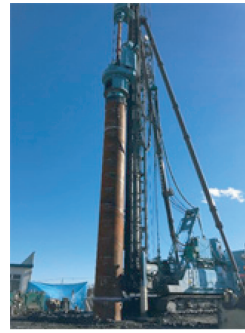
Photo 1 Kongo Pile™ method
