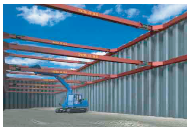
Fig. 3 Square steel pipe struts method
