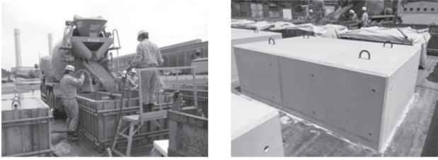
Fig. 4 Production of cuboid lump blocks
