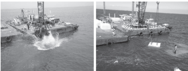
Fig. 7 Installation of stones and blocks
