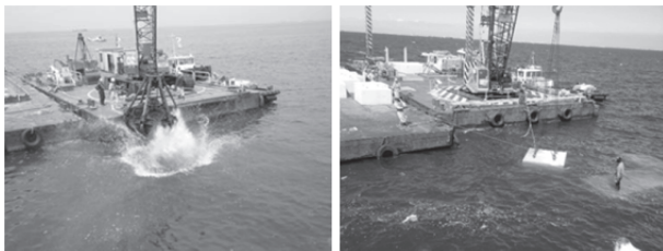
Fig. 7 Installation of stones and blocks
