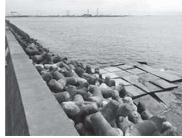
Fig. 8 Covering blocks (Ferroform blocks)
