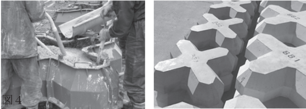
Fig. 5 Production of X-type blocks
