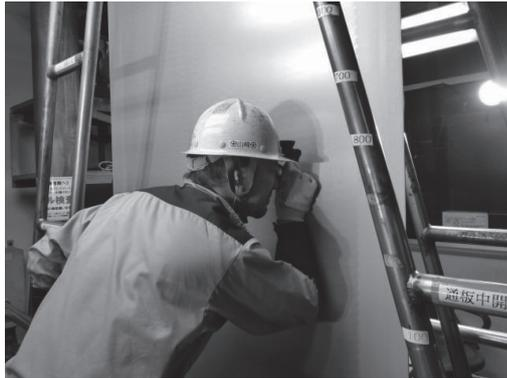
Photo 2 Inspection of scale defect
