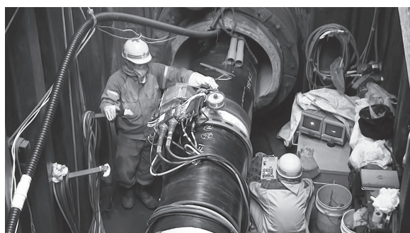
Photo 5 Appearance of pipe casing welding
