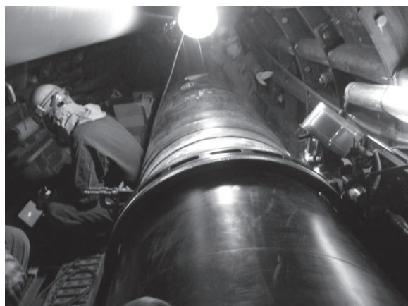
Photo 4 Appearance of welding in the shielded tunnel
