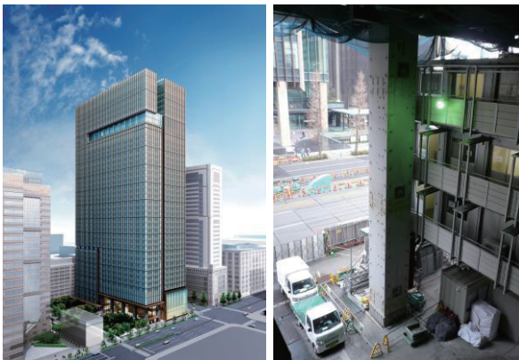
(a) Architectural rendering (b) Ultra-high strength concrete-filled welded box columns under construction
