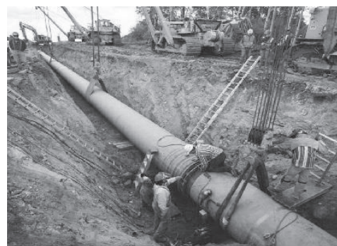
Photo 2 Construction Scenery of long distance pipeline used X100 grade linepipes
