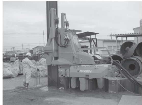
Photo 2 Piling by silent piler
