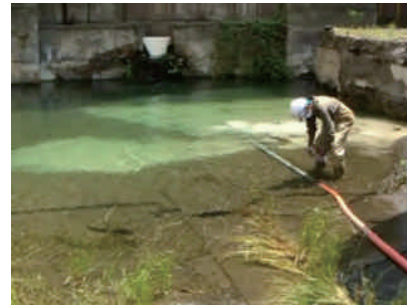
Photo 6 Casting in water
