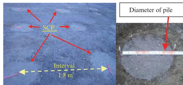
Photo 3 View of compaction pile (No. 4 Converter slag)
