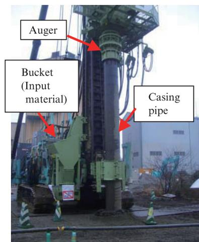
Photo 1 A view of construction examination
