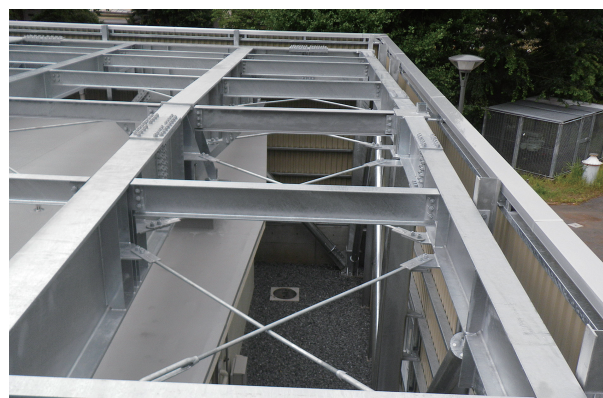
Photo 3 Governor station after reinforcement work (Roof)
