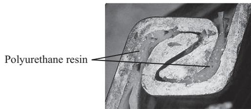
Photo 2 Previous waterproofing of steel sheet pile joints
