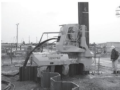
Photo 5 Installation by silent piler
