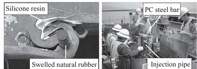
Photo 4 Picture and injection of silicone resin
