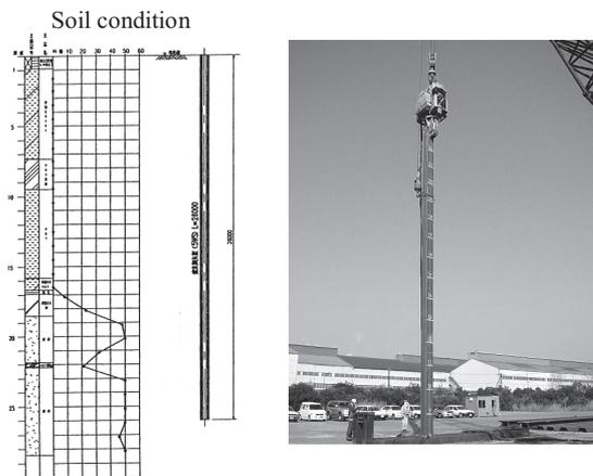
Fig. 6 Installation of long “J pocket pile”
