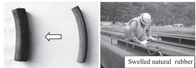
Photo 3 Picture and installation of swelled natural rubber
