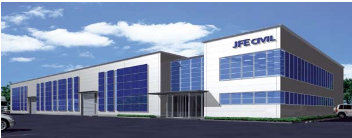
(c) Ecology grade applying photovoltaic generation system
