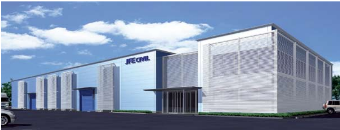
(b) Ecology grade applying louver
