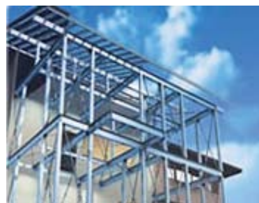
(1) Structural post and beam for residence
