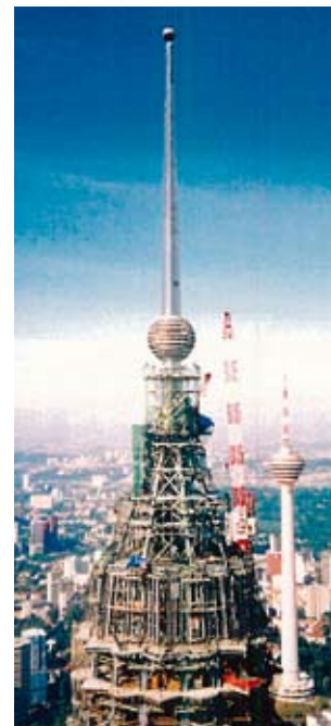
Photo 2 Lift up construction finished
