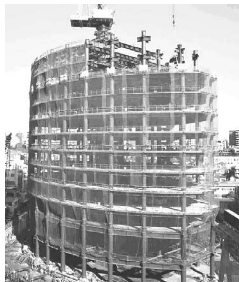
Photo 1 Example of building using circular columns
