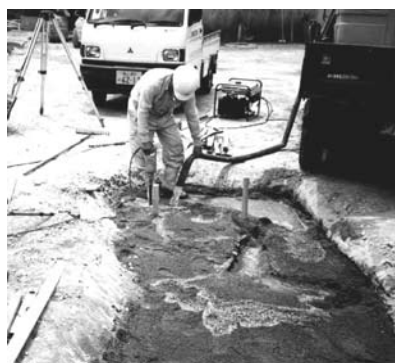
Photo 2 Experiment work (Hydraulic filling at second layer)
