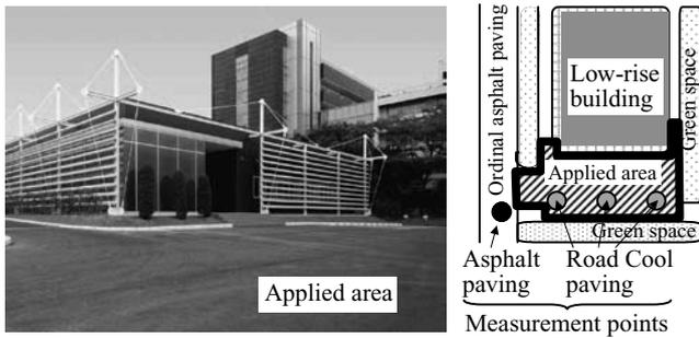
Fig.2 Schematic overview of temperature measurement of water retentive pavement using Road Cool
