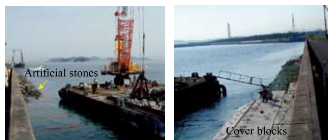
Installation of artificial stones
