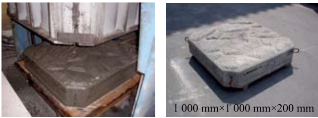
Forming After steam curing Photo 3 Production of Ferroform blocks for seawall
