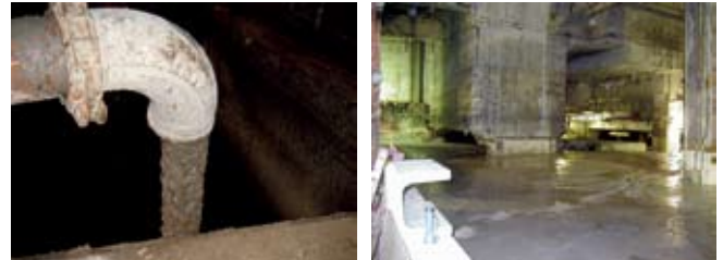
placing by concrete pump On placing Photo 5 Execution of fill in the basement by using fresh Ferroform
