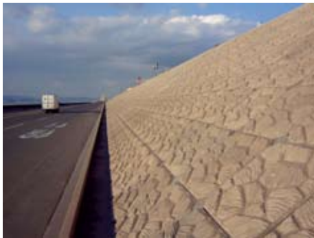
Photo 4 After completion of seawall construction using Ferroform blocks
