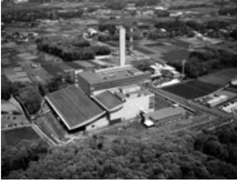
Photo 1 A view of Tobu Clean Center
