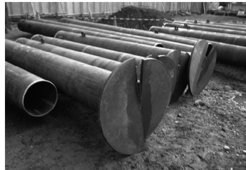
Photo 1 Screw pile, Tsubasa Pile
