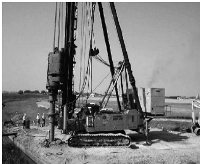
Photo 3 Construction of Tsubasa Pile using pile driver
