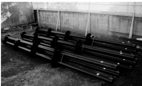
Photo 4 Screw pile, "Micro-pile with Plural Wings"
