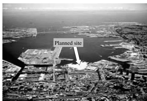
Photo 1 Port of Yokohama and planned site for Yamanouchi District Development Project
