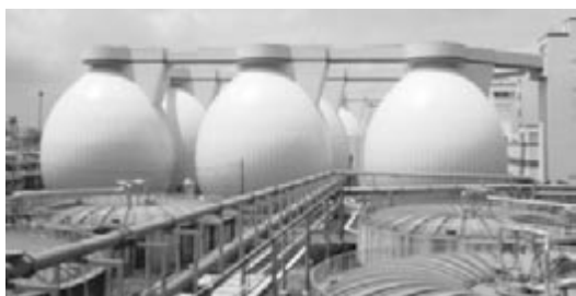
Photo 6 Egg-shaped digestion system for sewerage sludge
