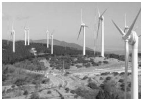
Photo8 Wind power generating equipments (2 types; 750 kW, 2 000 kW)
