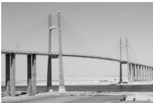
Photo7 Bridge over Suez Canal (Inclined drawbridge)
