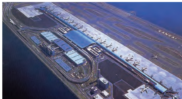
Example of application of JFE30-2 to roof (Kansai International Airport Terminal Building)
