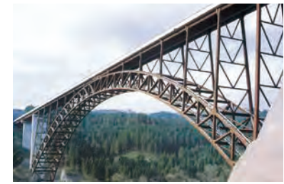
Appearance of bridge using weathering steel developed by JFE Steel
