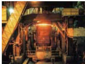
Ladle refining equipment
