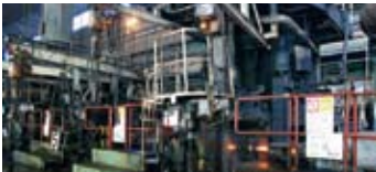
Rough rolling mill
