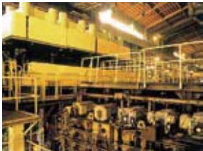
Continuous casting equipment
