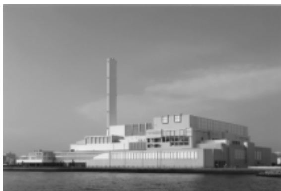
Photo 1 Kanazawa waste incineration plant in Yokohama city
