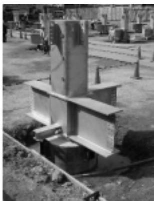
Photo 14 Column-to-pile joint
