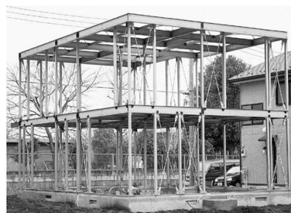
Photo 16 Steel frame of NKK-Frame Kit
