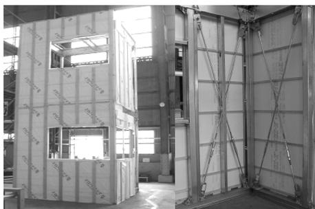
Photo 17 Insulation system of NKK-Frame Kit
