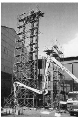
Photo 13 Construction test of CFT
