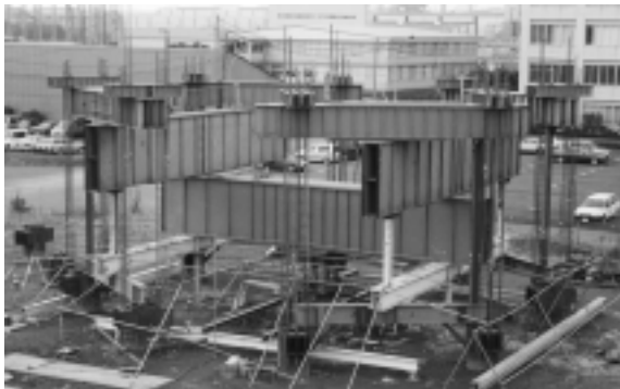
Photo 2 Static load test (d=1200mm)
