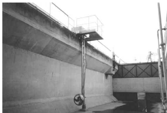
Photo 1 Oscillating mixer installed in anaerobic reaction tank at A-wastewater treatment center
