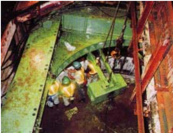
Photo 2 Ring erection under a street
