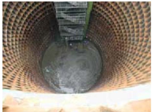
Photo 4 Finished bottom-slab concrete
