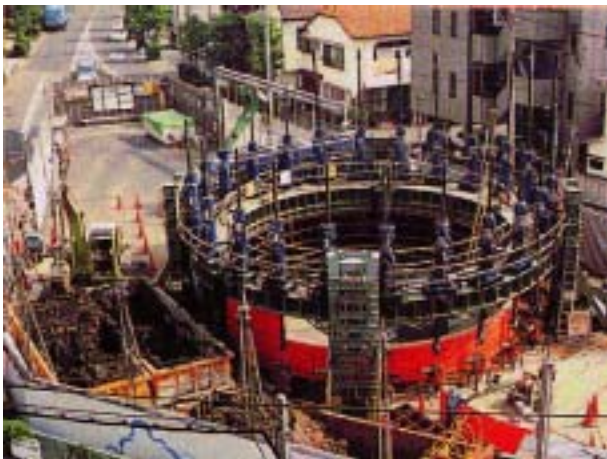
Photo 3 Scenery of large diameter "Urban-Ring" construction
