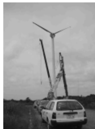
Photo 9 Installation of LW50/750 wind turbine (Esashi)
