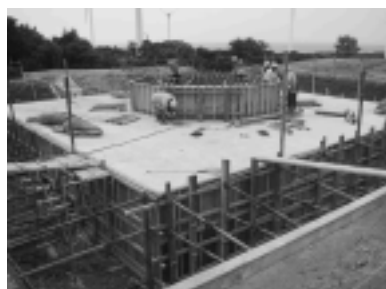
Photo 5 Construction of foundation w/RC pile (Esashi)
