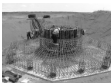
Photo 6 Construction of foundation w/steel pile (Horonobe)
