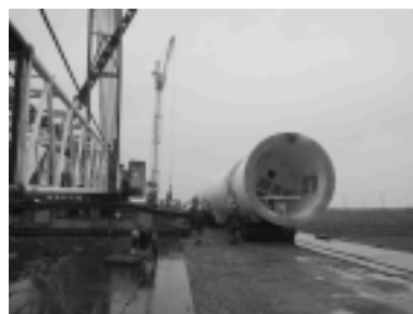
Photo 4 Carrying of tower block into site (Horonobe)
