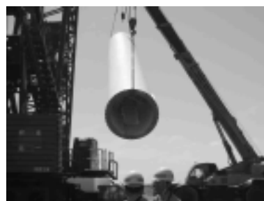
Photo 7 Lifting of tower bottom block by 350t crane (Horonobe)
