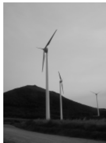
Photo 1 LW50/750 w/hub height 74m towers (Esashi)
