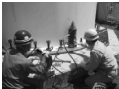
Photo 2 Tightening of PC anchor bolt by hydraulic Jack (Horonobe)
