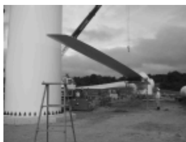
Photo 8 Setting of rotor & blades on ground (Esashi)
