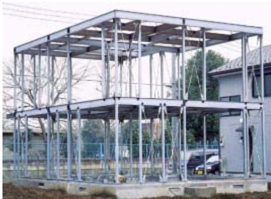
Photo 1 Frame with braced panels
