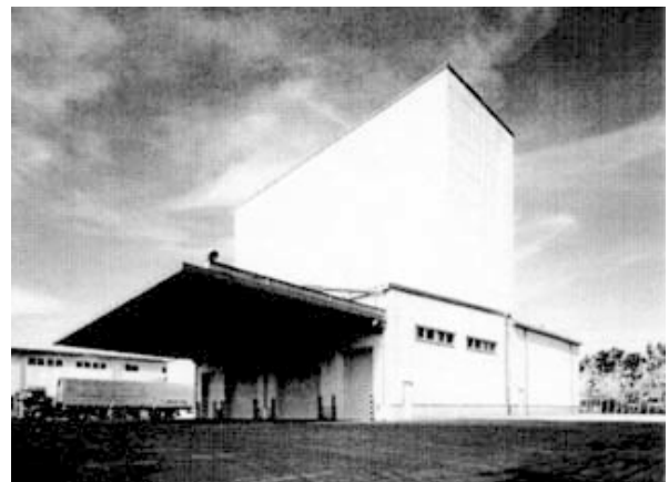
Photo 1 Appearance of the racking with roof and wall
