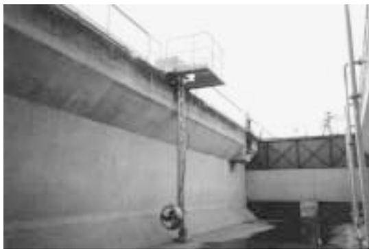
Photo 3 Oscillating mixer installed in anaerobic reaction tank at A-waste water treatment center
