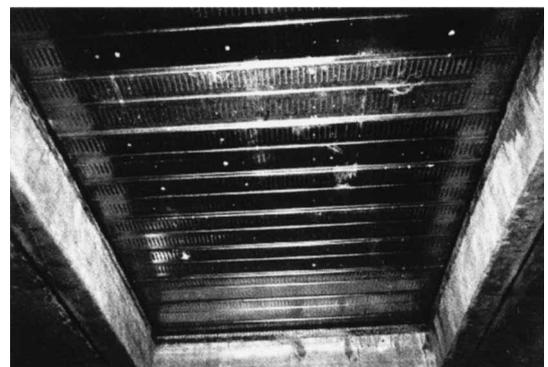
Photo 1 Under view of concrete slab using Hi-Deck R-100
