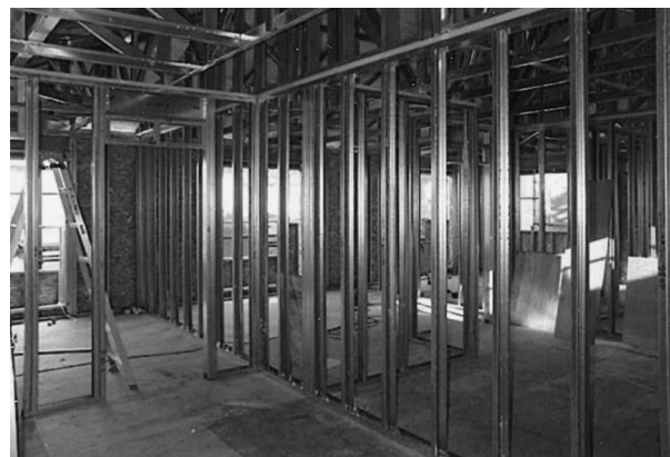
Photo 2 Light-gauge steel structure of an apartment house in Funabashi city
