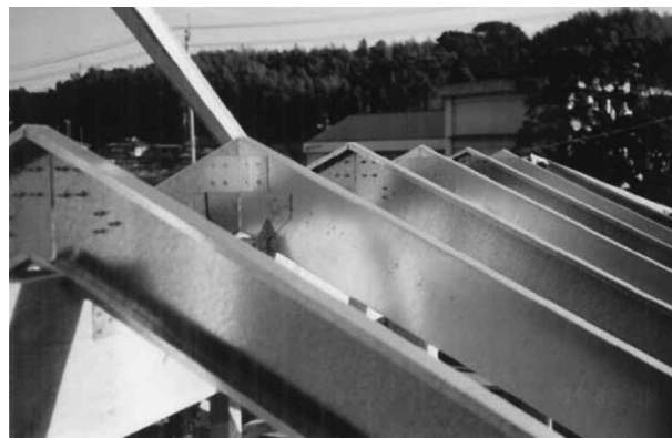
Photo 4 Light-gauge steel rafters for conventional wooden house
