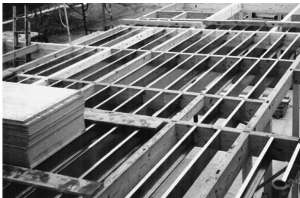
Photo 3 Light-gauge steel joists at 2nd floor for conventional wooden house
