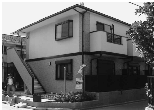
Photo 1 Apartment house using light-gauge steel shapes in Funabashi city
