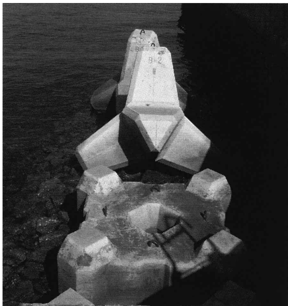
Photo 1 Breakwater blocks and cover blocks of Ferroform at Mizushima Port (Exposure from February, 2000)
