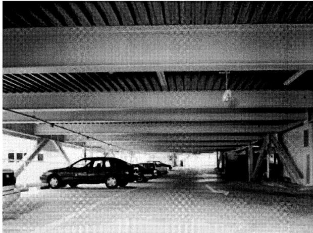
Photo 1 Building for mobile car park using fire resistant steel
